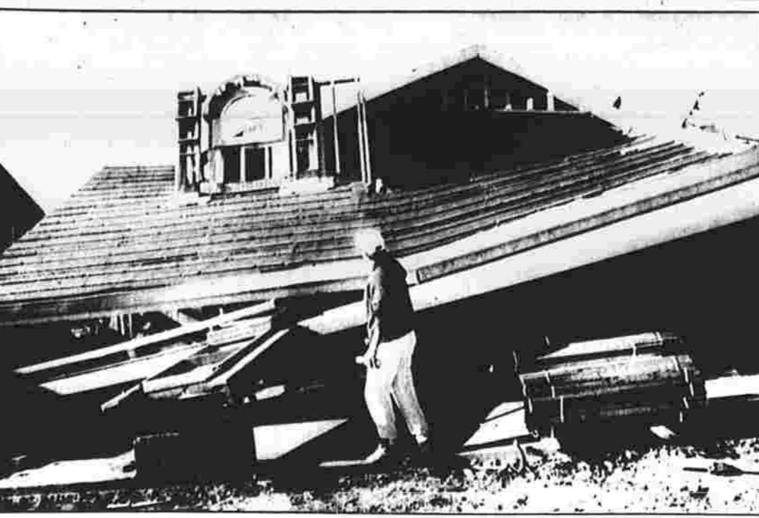
HIGH WINDS — Patrick Lyons, a worker for a housing development in Fairfield, Calif., looks over a home under construction that was wrecked by heavy winds Thursday in northern California.
